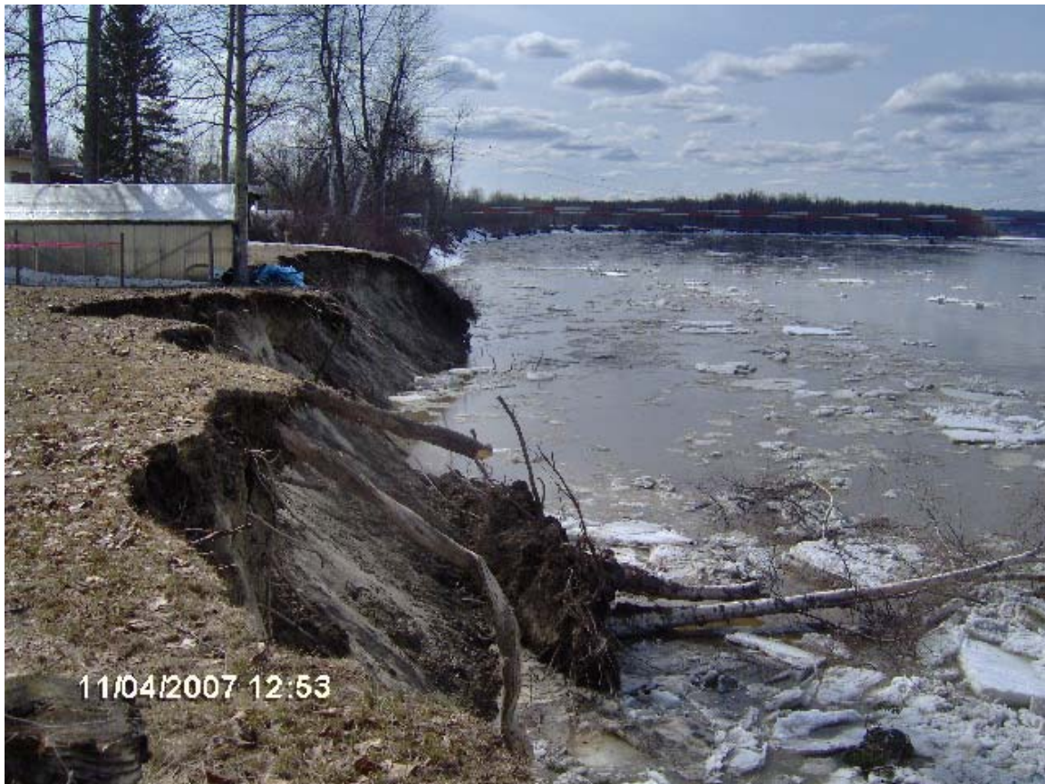
Figure 2 – Eroded Bank Prior to Stabilization Work
