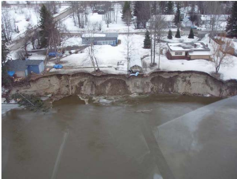
Figure 1 – Eroded Bank in Late March, 2007
