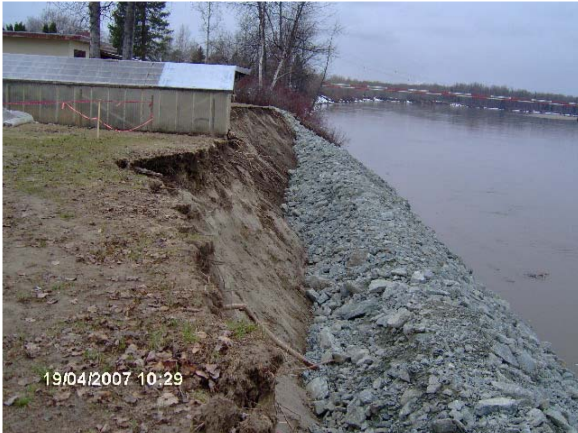
Figure 3 – Riprap Dyke After First Phase of Construction
