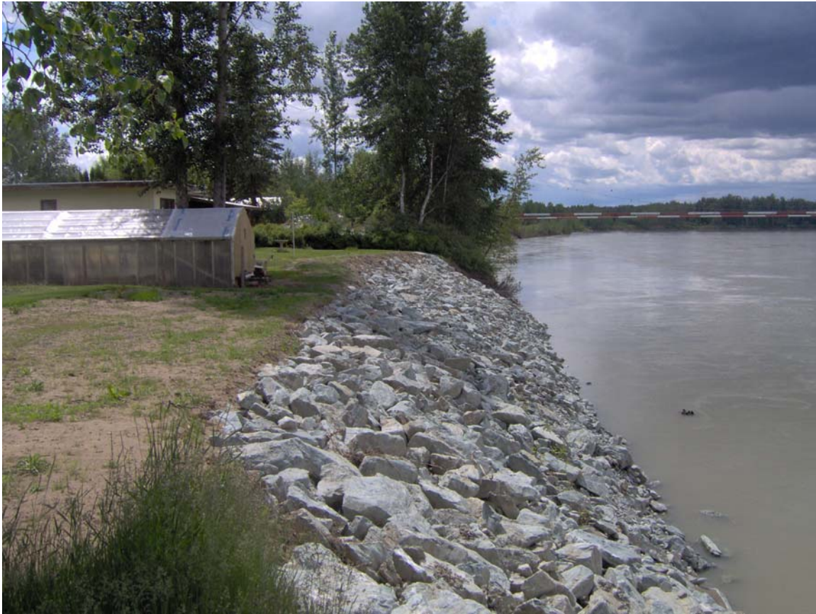
Figure 4 – Stabilized Bank at Shelley
