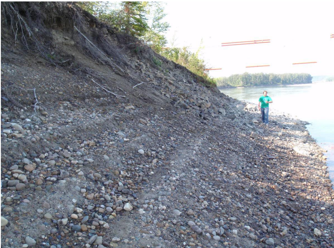
Plate 6. Downstream view showing remnants of previous riprap work within Spectra's ROW.
