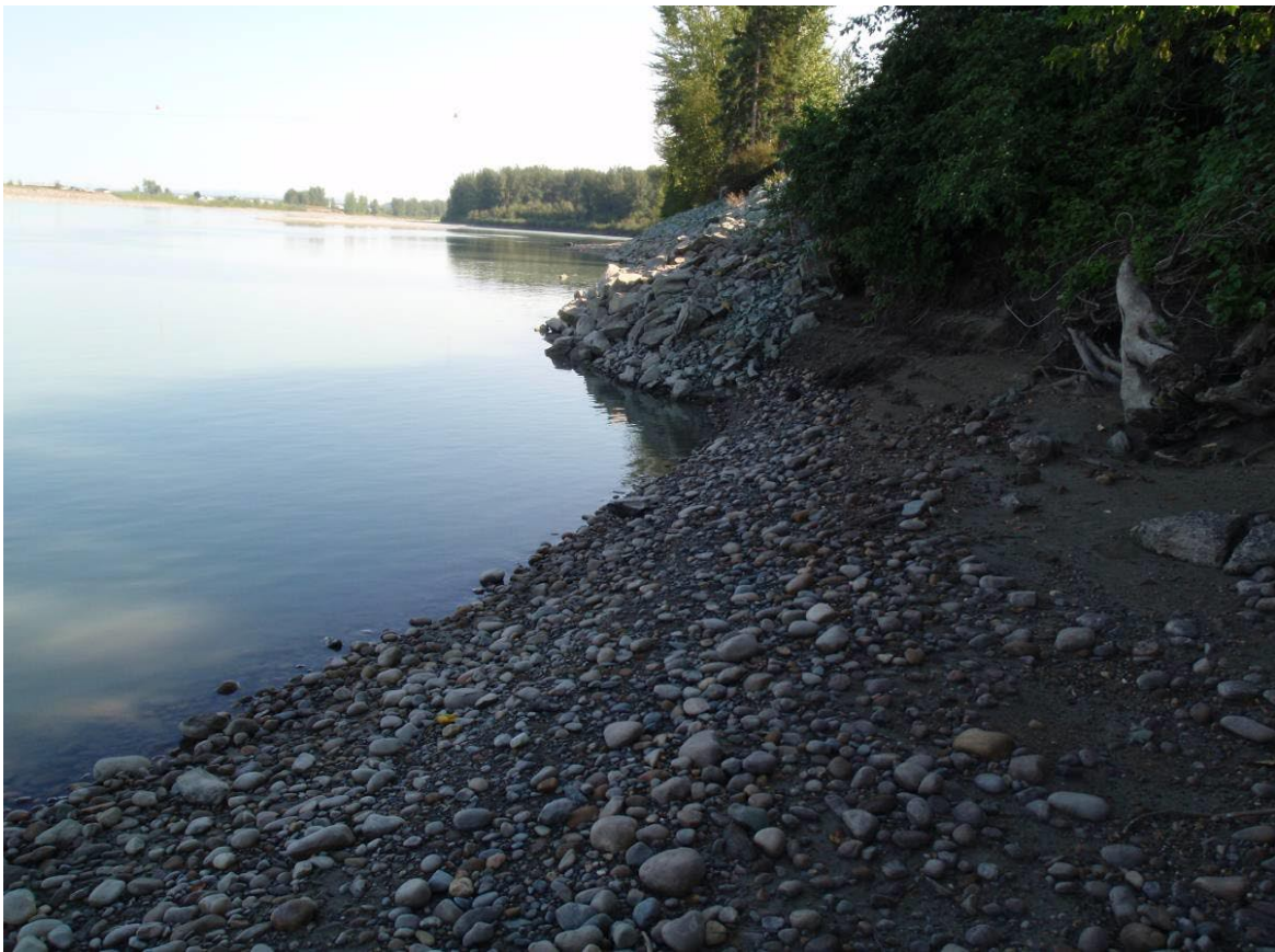
Plate 5. Upstream view showing the tie in point with the 2007 revetment project.
