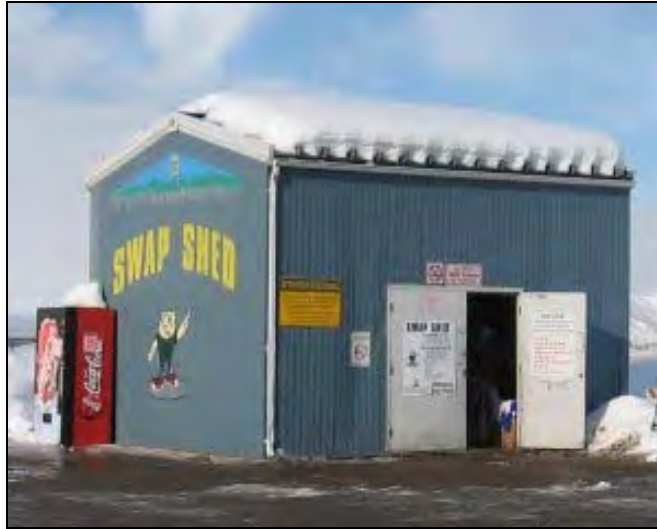
Figure 6. Swap Shed at Foothills Boulevard Regional Landfill
