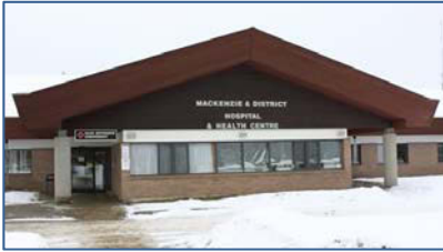
Mackenzie & District Hospital
